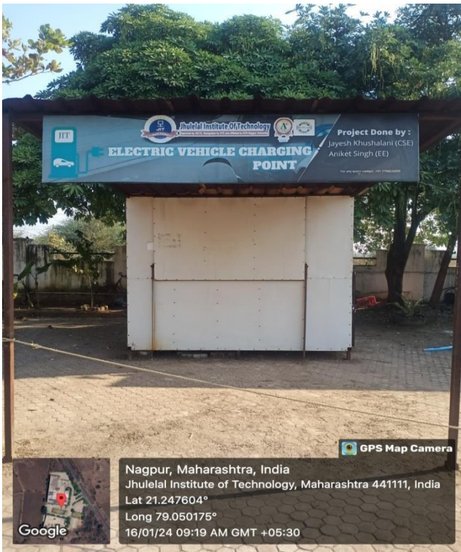
E-Vehicle Charging Point
